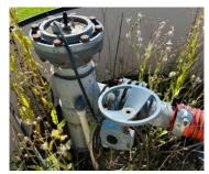
Addendum No. 1 RFP No. 322039 Site No. 2 Rodefeld Landfill (Site No. 2) – All gas wells have QED Wellheads. Visual valve positions are available. Additionally, some gas wells may have additional LOCI units installed.
