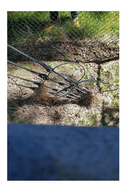
Typical guy wire. Guy wires to be removed flush with the ground surface. Surrounding fencing to be removed.
